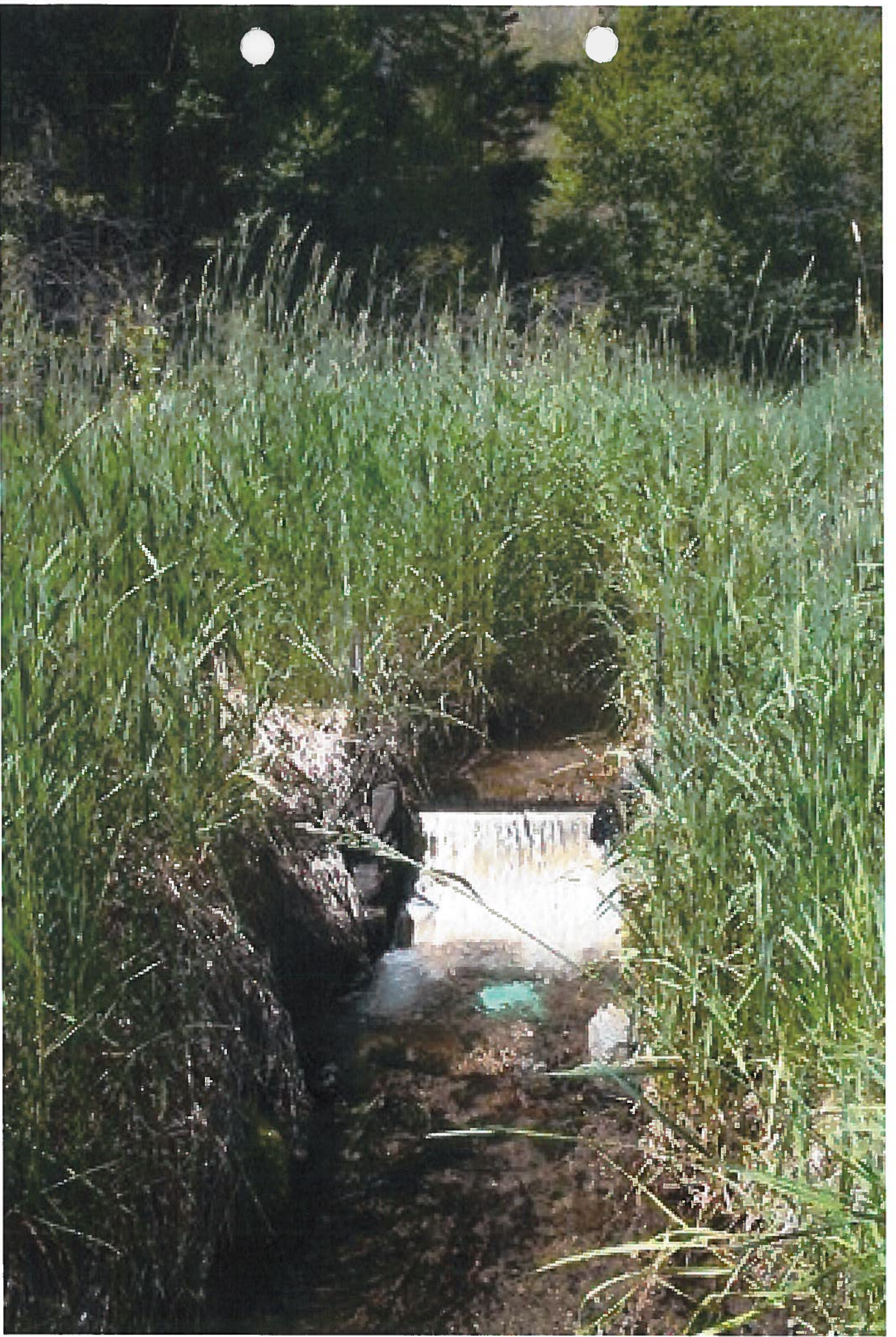
Coanda Screen diversion box, JPR
