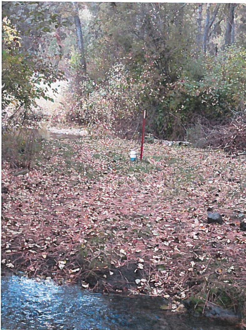
This looks upstream from the turbine house. Indian Creek is the water in the top half of the photo. The water at the bottom is the outflow from the turbine. The blue and white pipe near the fence post in the center is the valve for the turnoff.
