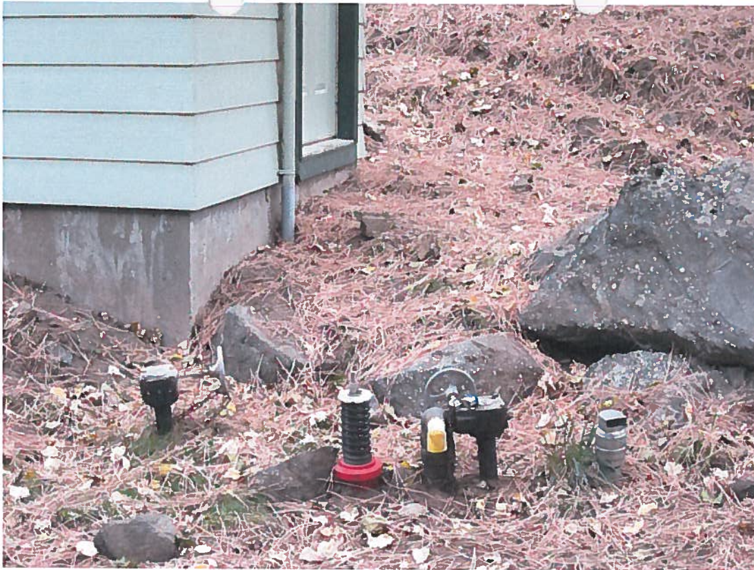
The irrigation system and the turbine share the same water supply. There is a re-diversion for irrigation at the turbine house.
