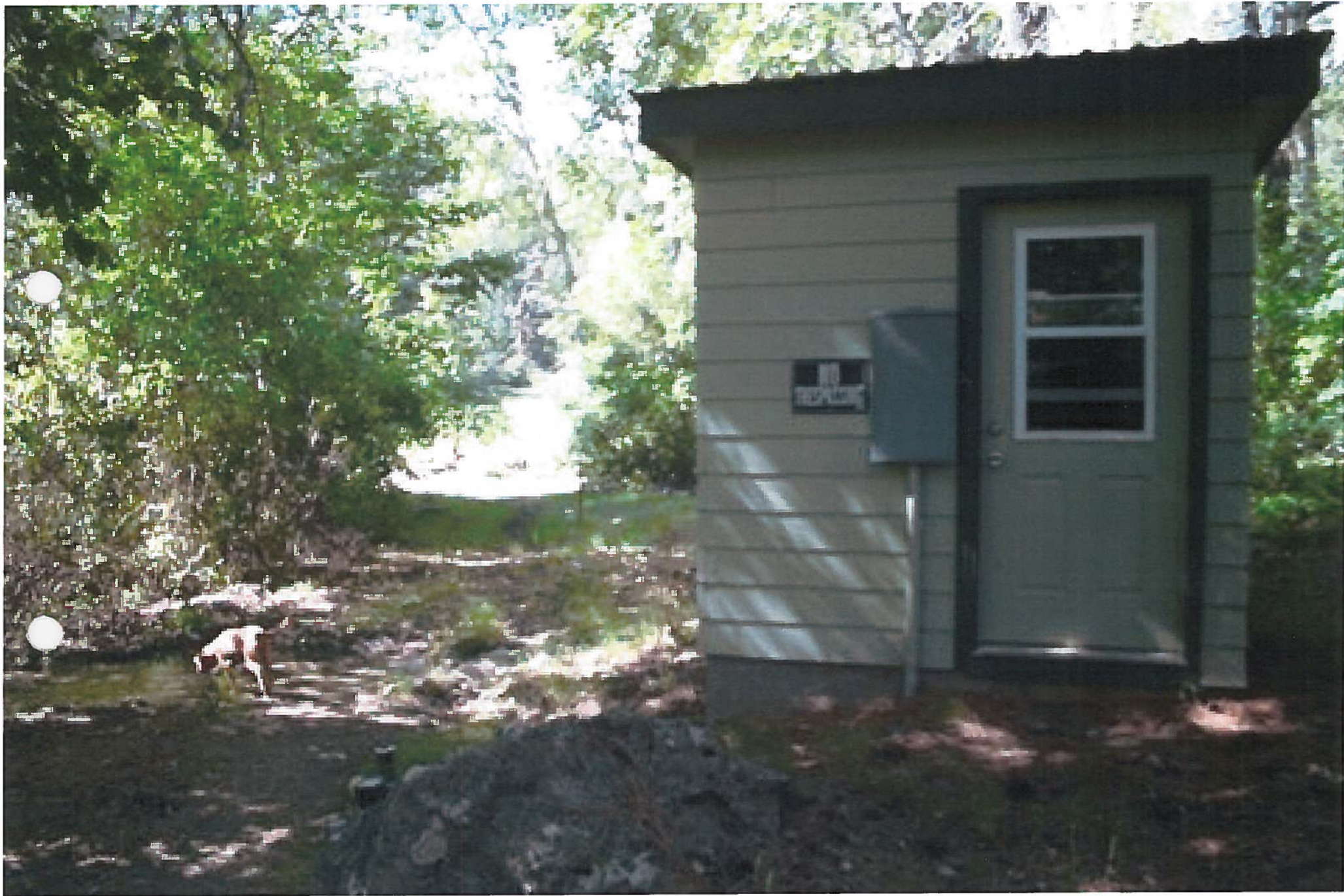
Turbine shed & discharge. JPG
