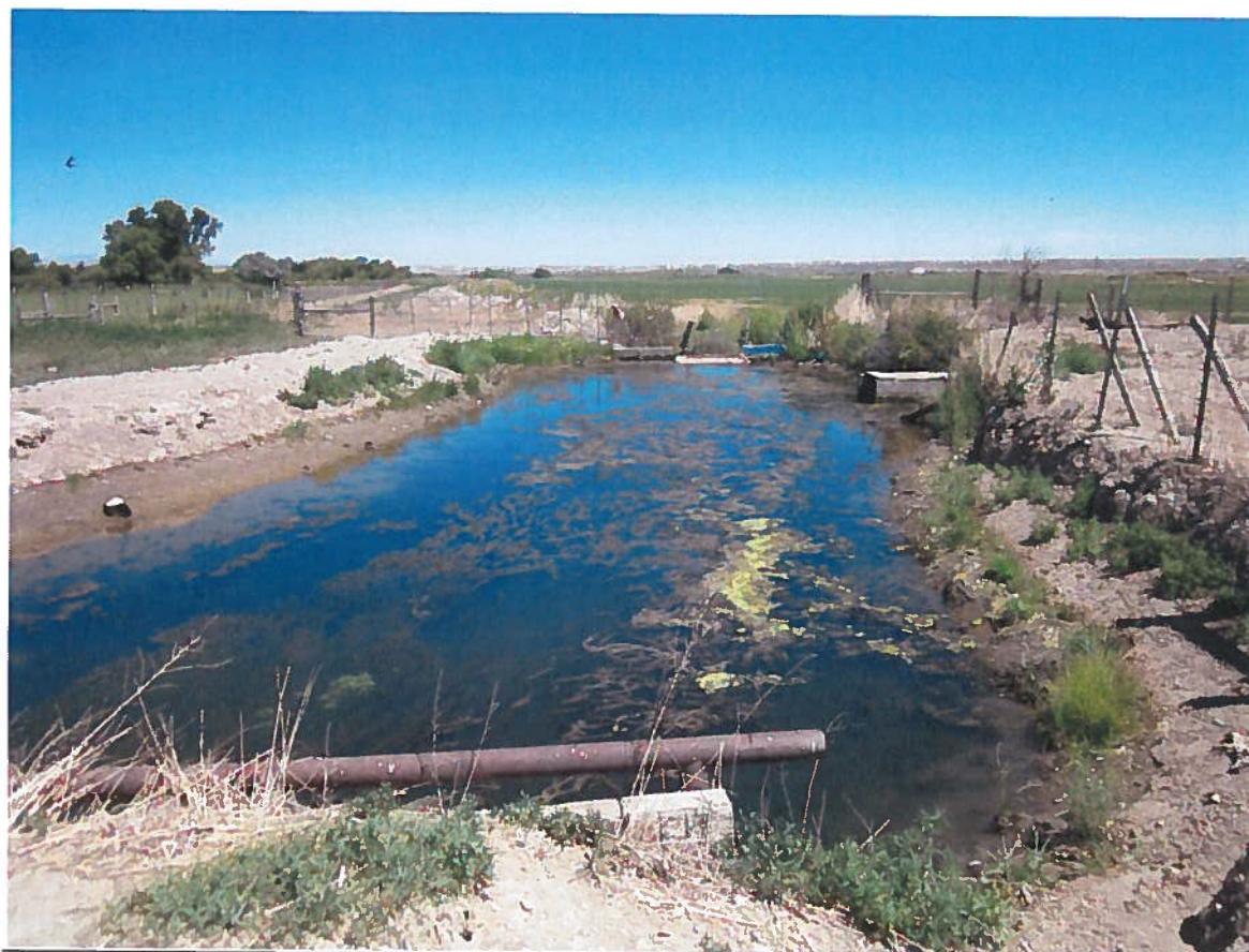
The image above shows flow through pond looking east. The concrete structure in the right upper-middle of the photograph is the headgate which diverts water to the pump.
