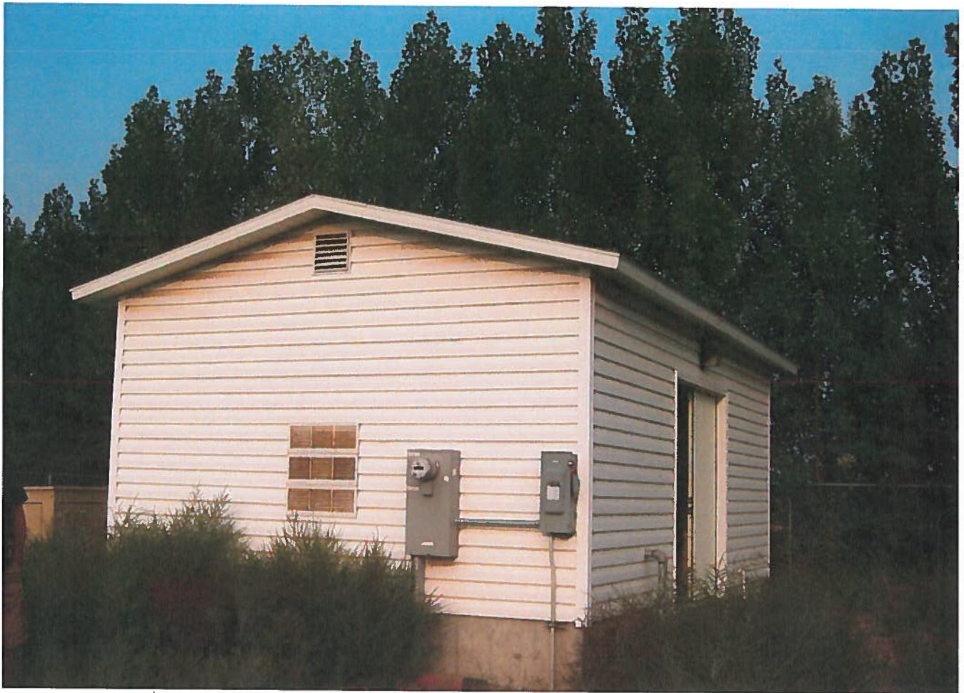
North well is inside wellhouse
