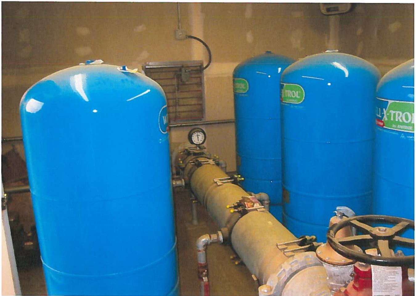
Inside north well house
