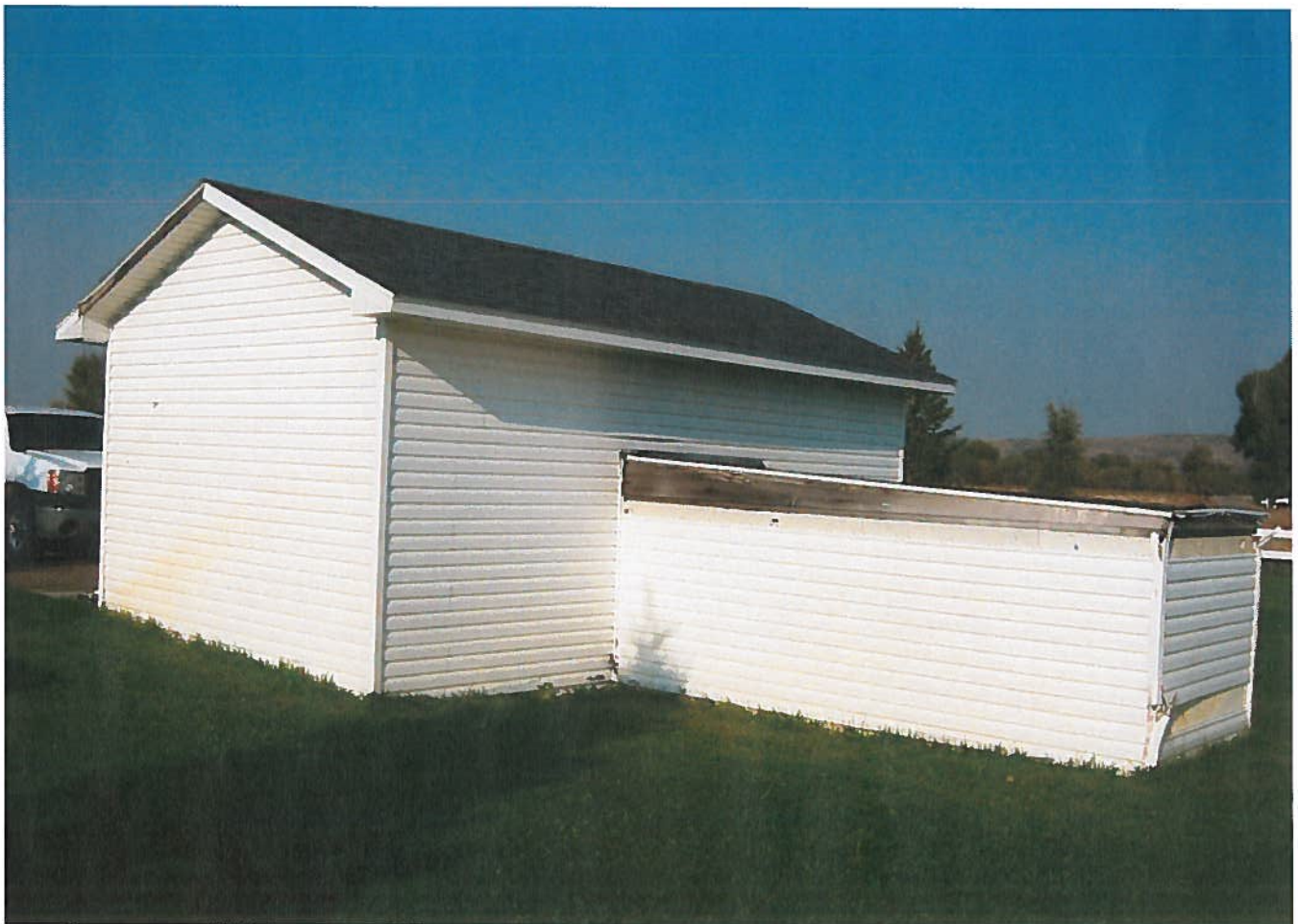
Well house - well is in short portion
