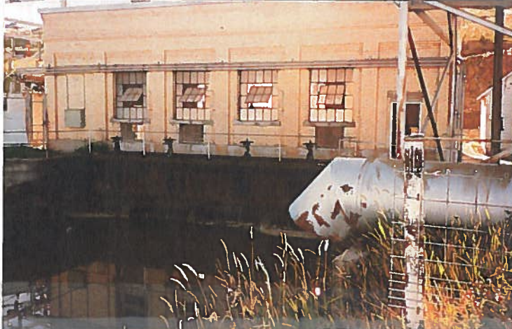
↗ waste water overflow
