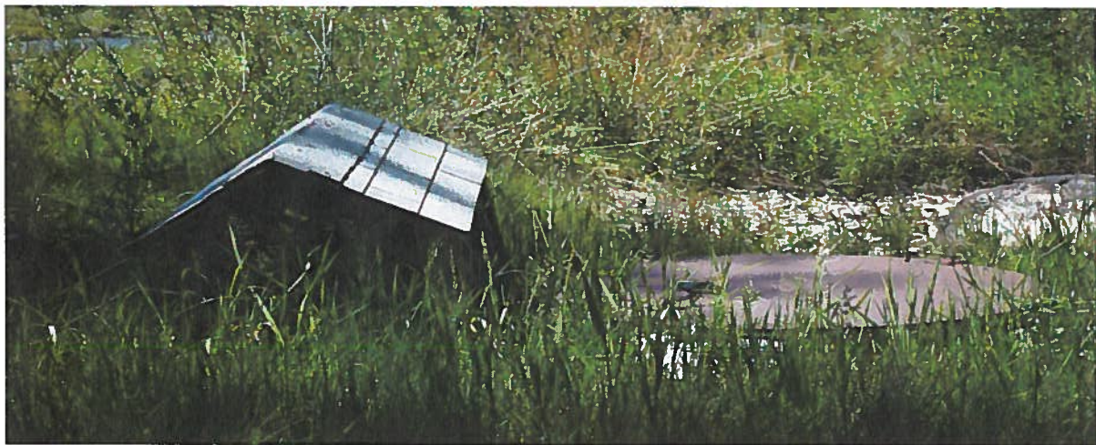
Pump and return flow tank
