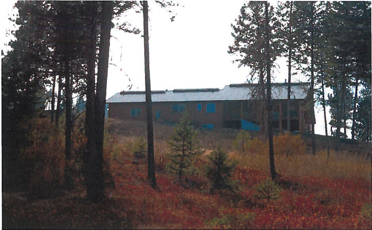
Place of Use: View westerly of a typical home located in the West Pine Subdivision. The fire protection system serves 60 residential lots within the West Pine Subdivision.
