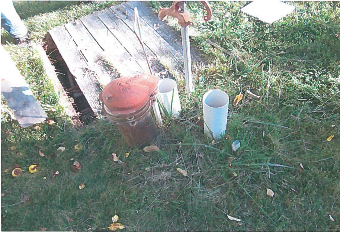
6" diameter well located southwest of the house.
