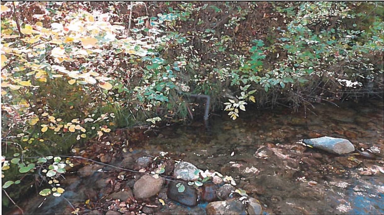
Point of Diversion: View southwesterly of a 1 1/2" steel pipe screened suction line in Warm Springs Creek. The right holder has constructed a small rock dam to create a pool for pumping.
