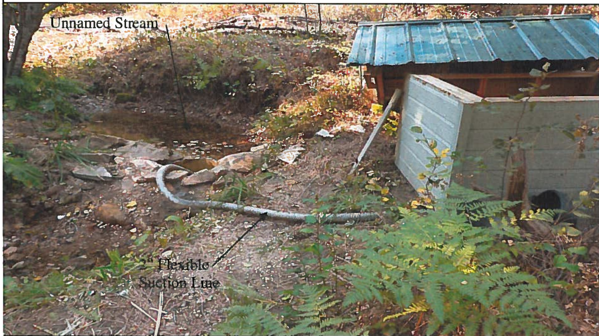
Point of Diversion: View westerly of 2" flexible suction pipe extending from pump enclosure box to 24" diameter PVC cistern or sump in unnamed stream.
