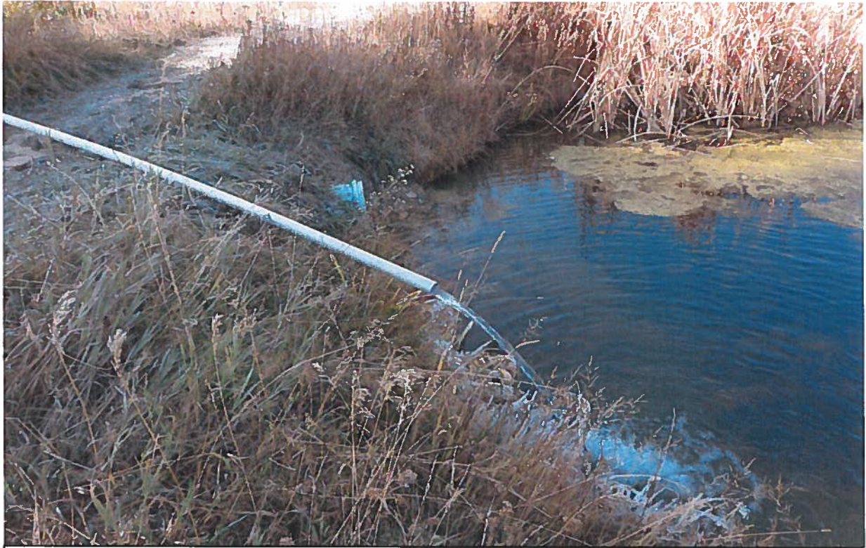
View southwesterly of the 1 ½" PVC pipe supply line discharging into a pond. Water is pumped from the pond for irrigation of the right holders lawn, landscaping, and gardens.
