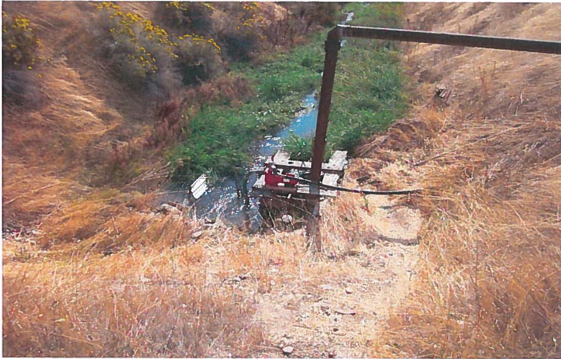
2 hp pump and 2" pipe from the unnamed ditch that runs along the east boundary of the Lyons property.
