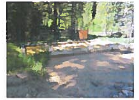
MIDDLE DRYING POND AND LOWER POND
