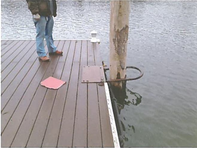
NE corner of dock and 1 1/4" discharge line
