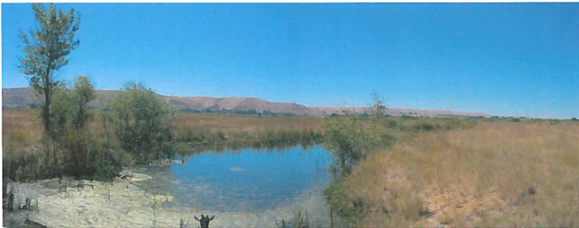
Standing surface water below HVAC discharge pipe. Photo taken looking west.
