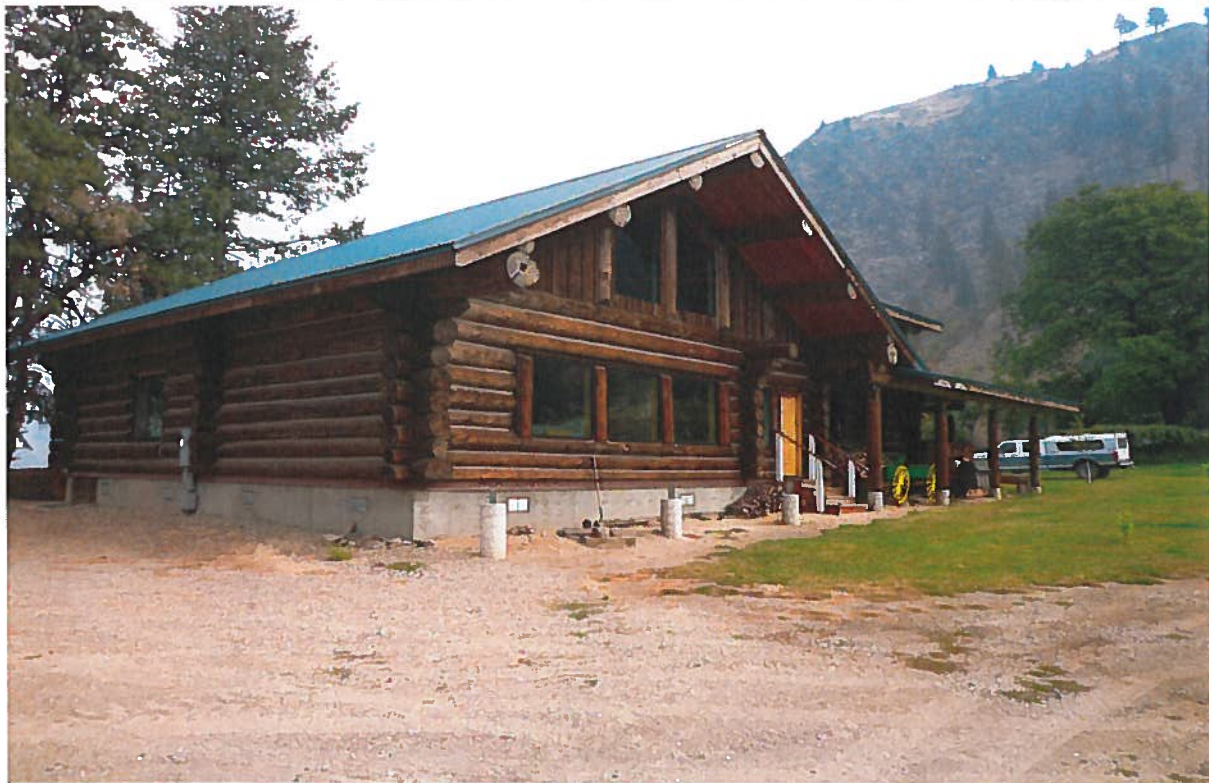
Place of Use: View northeasterly of the home served by the hydropower system.
