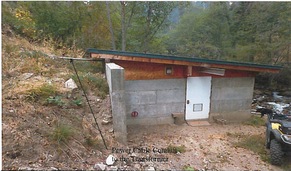
View southerly of the power station located approximately \frac{1}{2} mile downstream of the penstock inlet structure. The penstock size increases from 10" to 12" at the power station.
