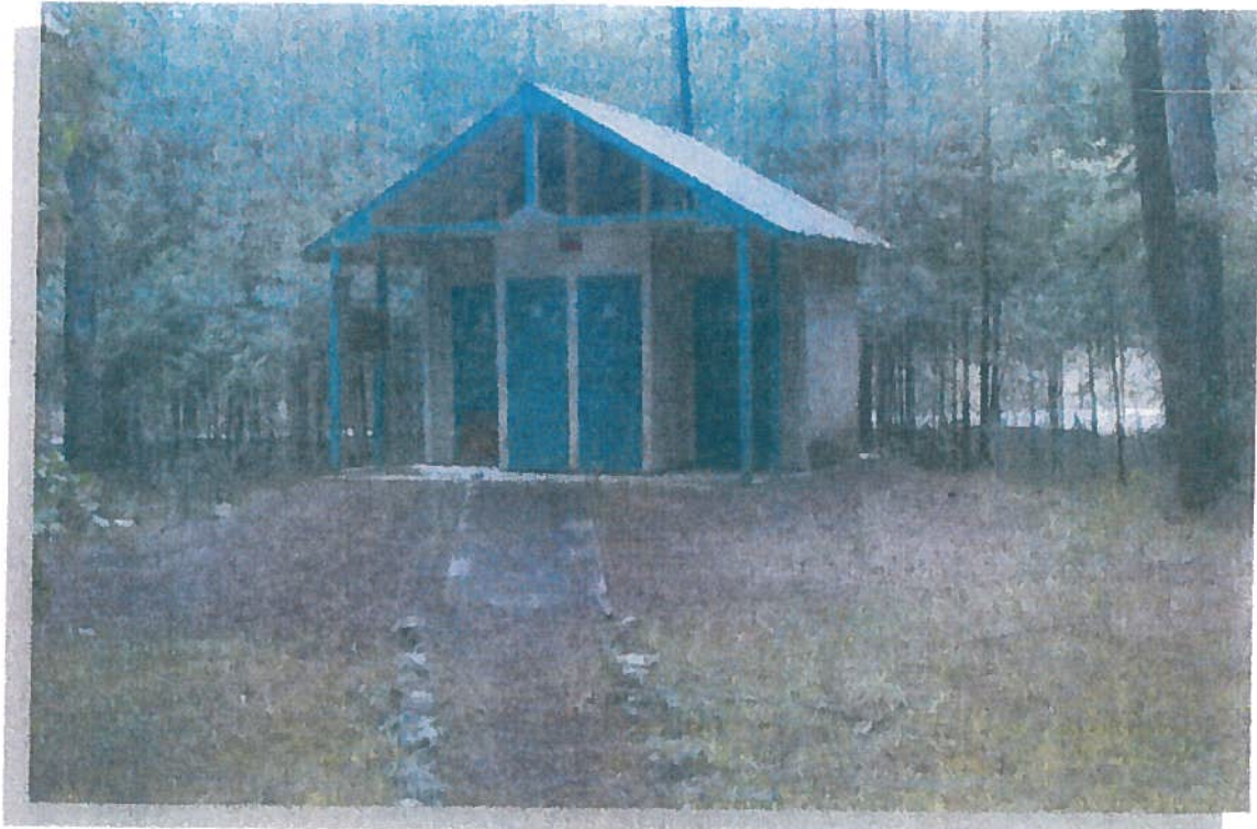
Concrete vaulted pit toilet — Bear Paw Campground, looking north.
