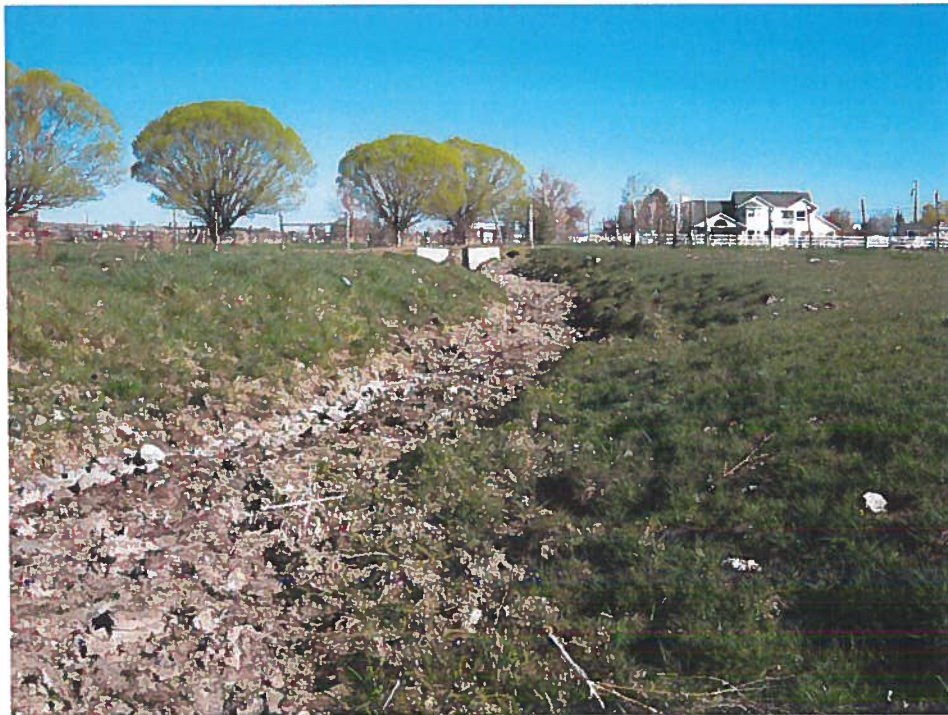
Figure 1: View of pond looking NW towards check dam.
