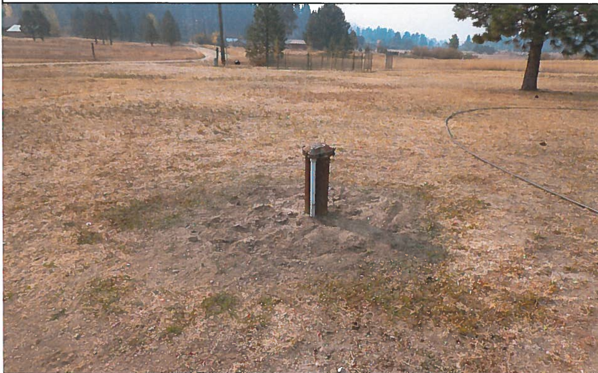
Point of Diversion: View southerly of ground water well located southerly of home.
