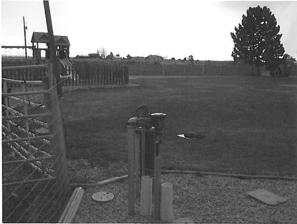
63-33200 Exam 3/21/2013: P/D well with portion of lawn and automated sprinkler irrigated field in background facing southeast.
