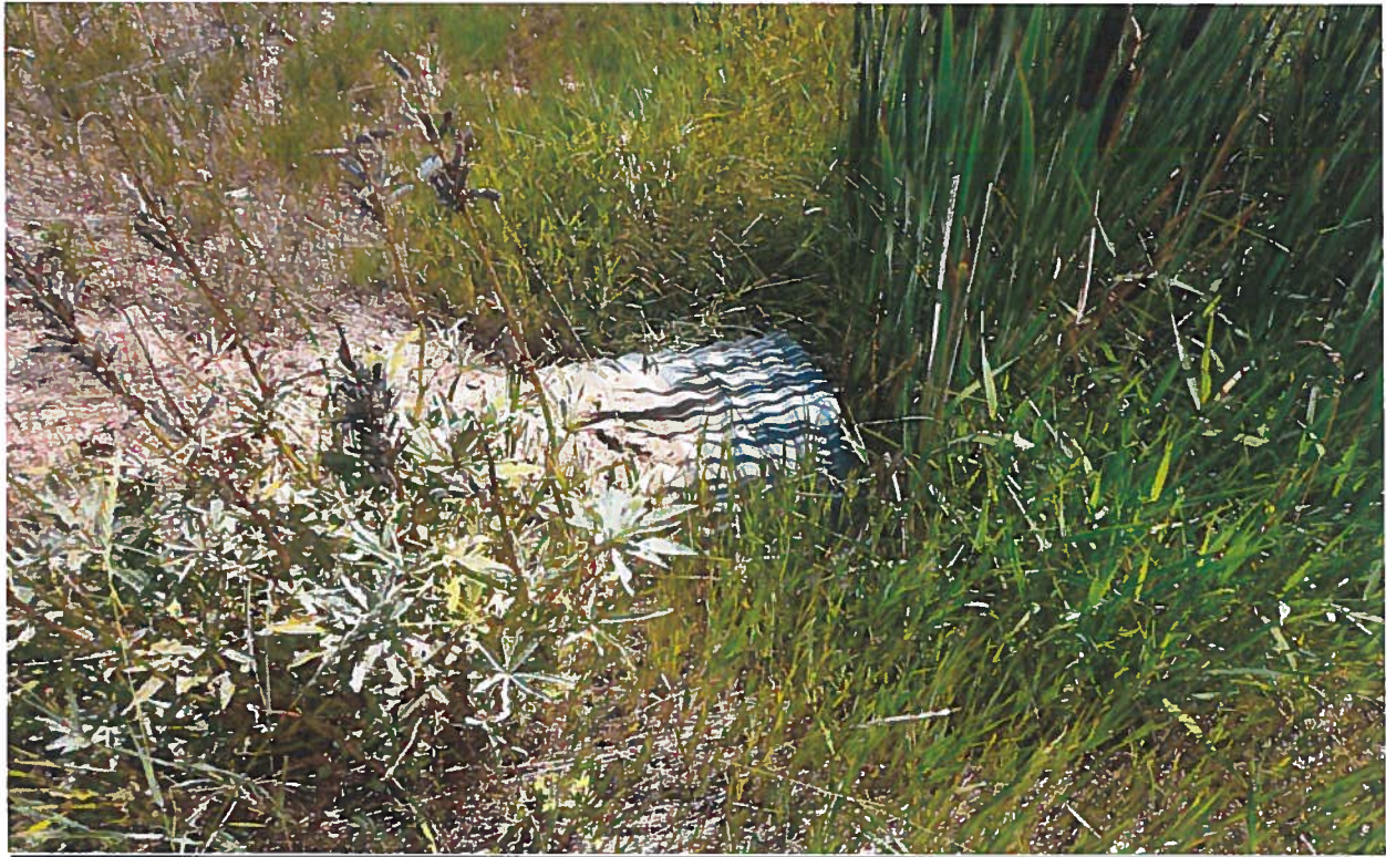
View easterly from the dam of the 36" CMP storage pond spillway. The storage pond overflow discharges downstream to the unnamed stream.
