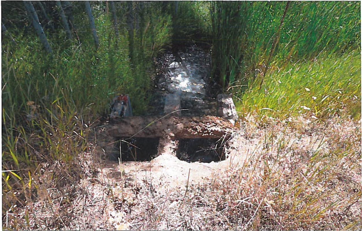
View southerly of aesthetic and wildlife storage pond concrete spillway. The two concrete spillway channels discharge water to a small section of the unnamed stream before discharging to the Ramos' storage pond to the south.
