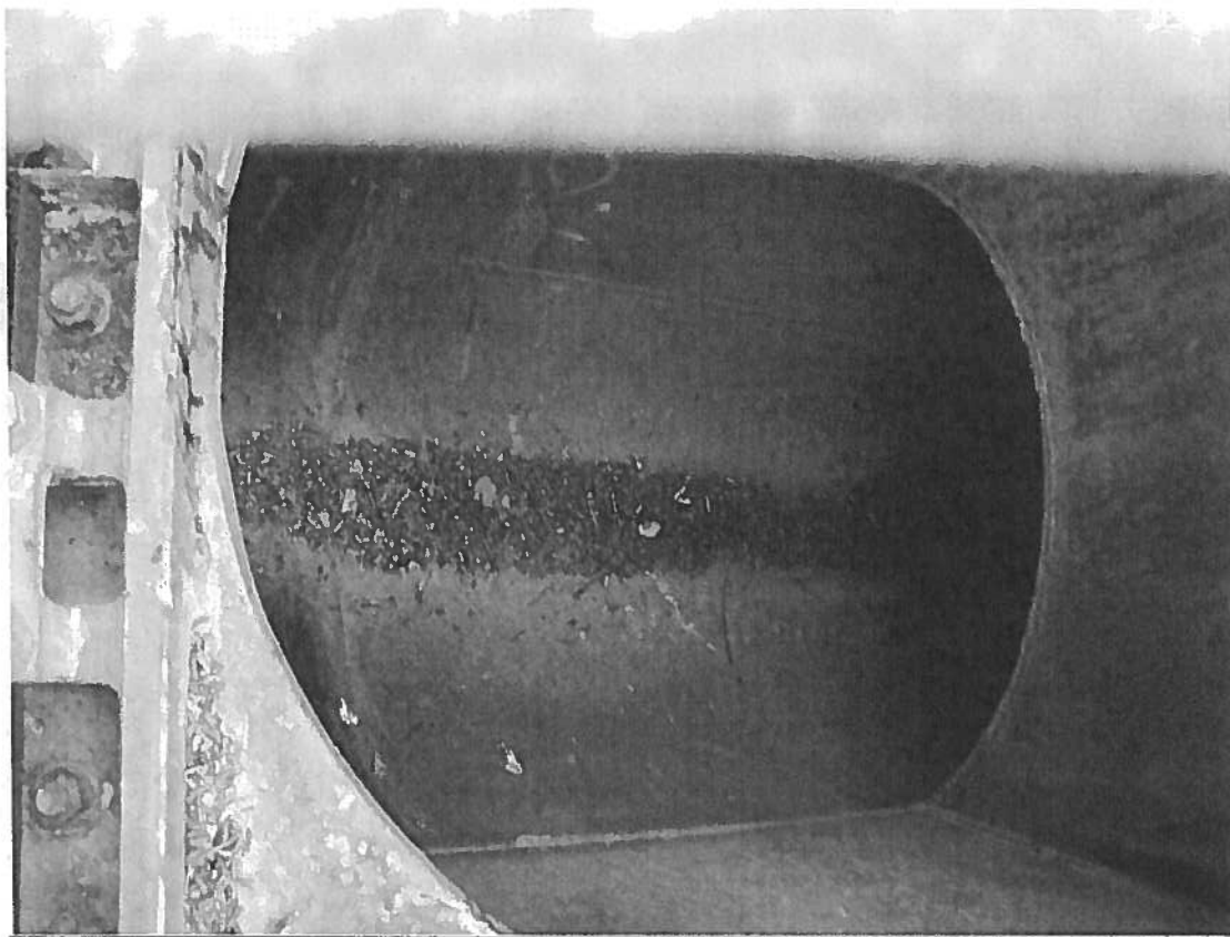
Photo of drop inlet transition from gate to pipe.
