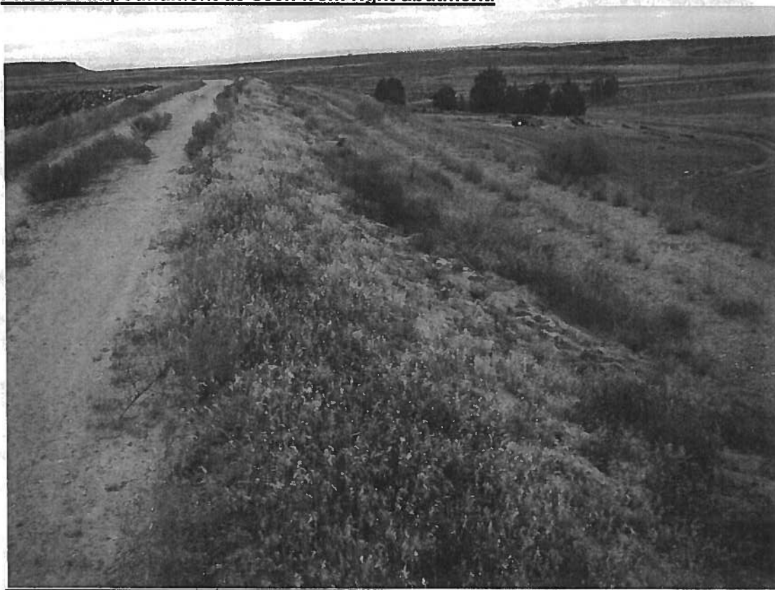
Photo of crest and downstream face viewing growth on embankment faces.
