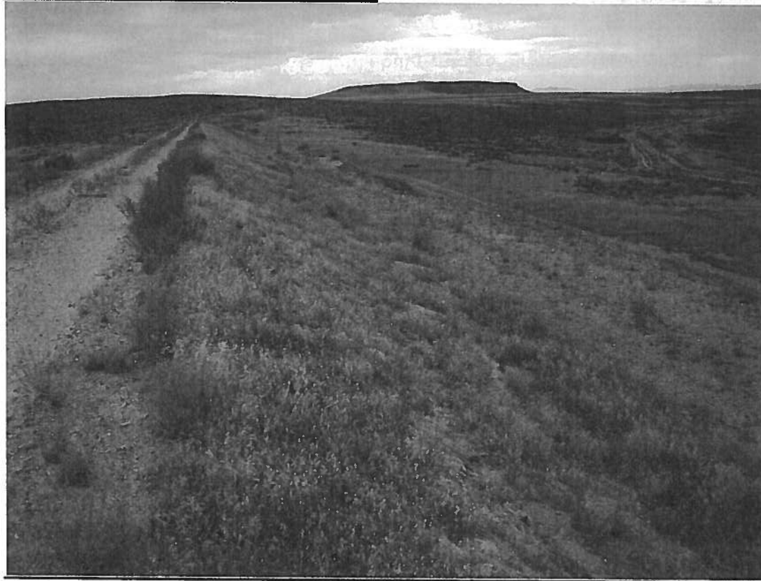
Photo looking towards left abutment downstream slope of embankment.
