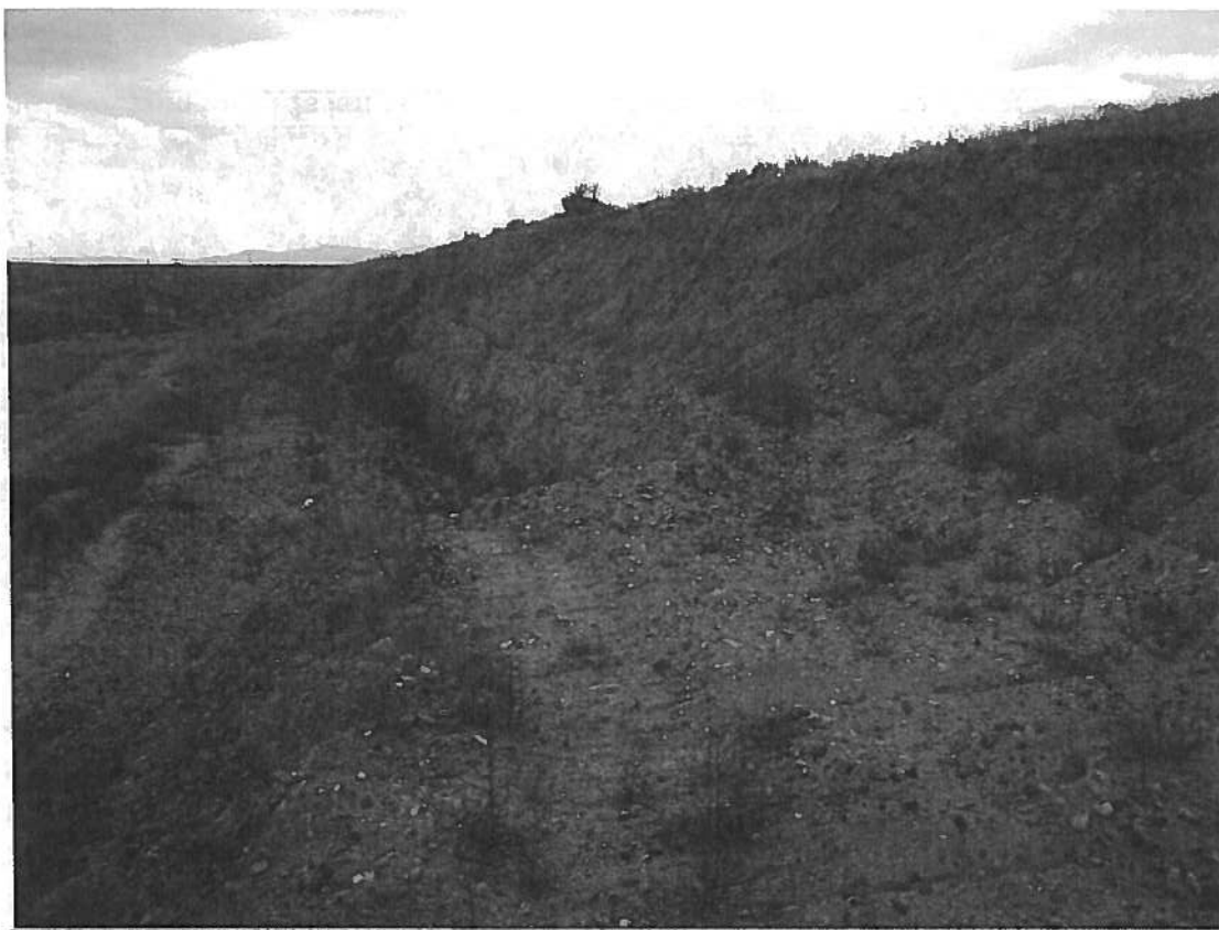
Photo looking southerly towards right abutment at area where removal of embankment material has been excavated.
