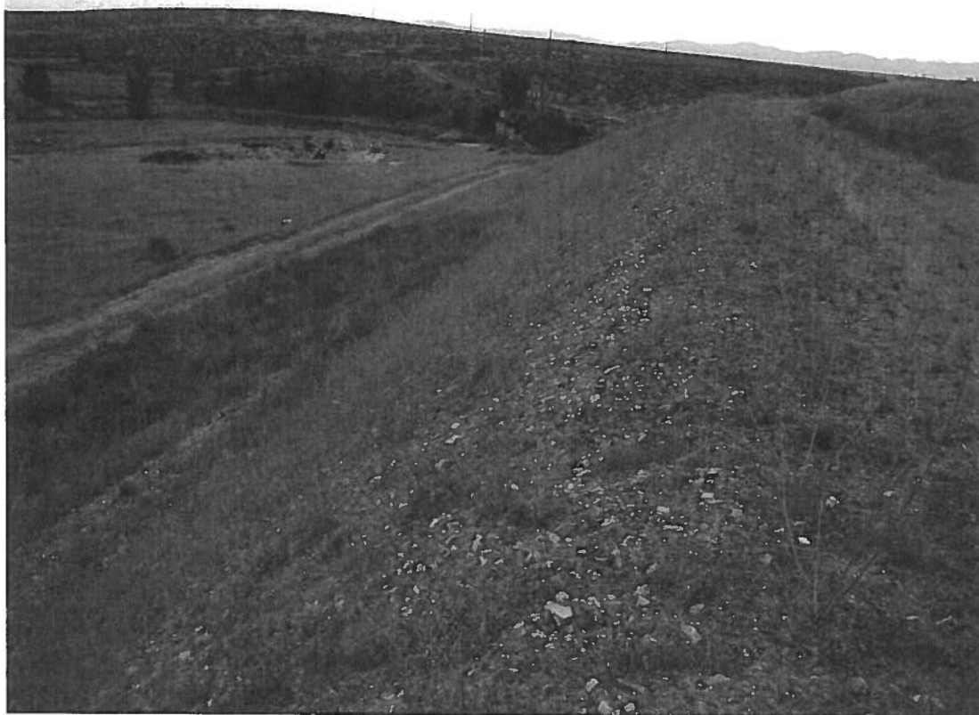
Photo viewing downstream face of dam as viewed from mid way point on dam looking towards right abutment.
