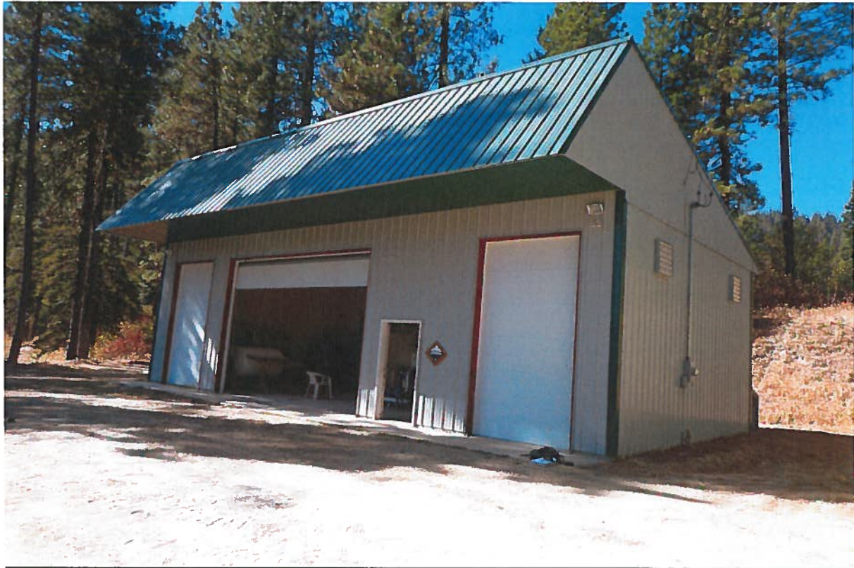
View westerly of the water treatment plant.
