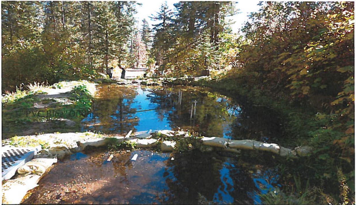
View easterly of the settling/filter pond. The six (6) 1" PVC vertical pipe sections are used to blow sediment out of the 4" PVC collection lines located around the perimeter of the filter section of the pond. Water is diverted through six (6) filtered perforated pipe sections connected to the 4" collection lines.
