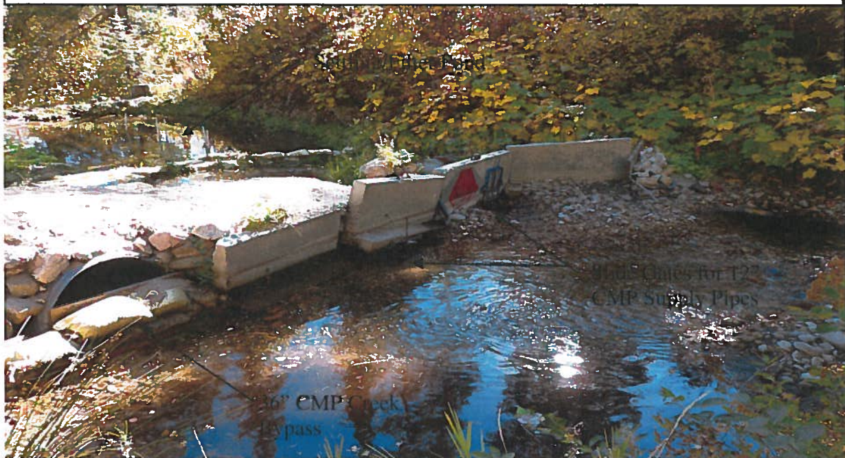
Point of Diversion: View southeasterly of concrete and earth dam on Warm Springs Creek. Three (3) 12" CMP pipes, two controlled by slide gates, diverts water from Warm Springs Creek to a settling/filter pond shown downgrade of dam.
