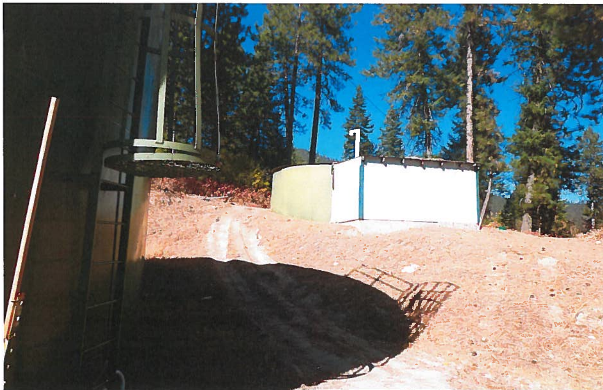
View northwesterly of the 40,000 gallon water storage tank located upgrade of the 100,000 gallon water storage tank.
