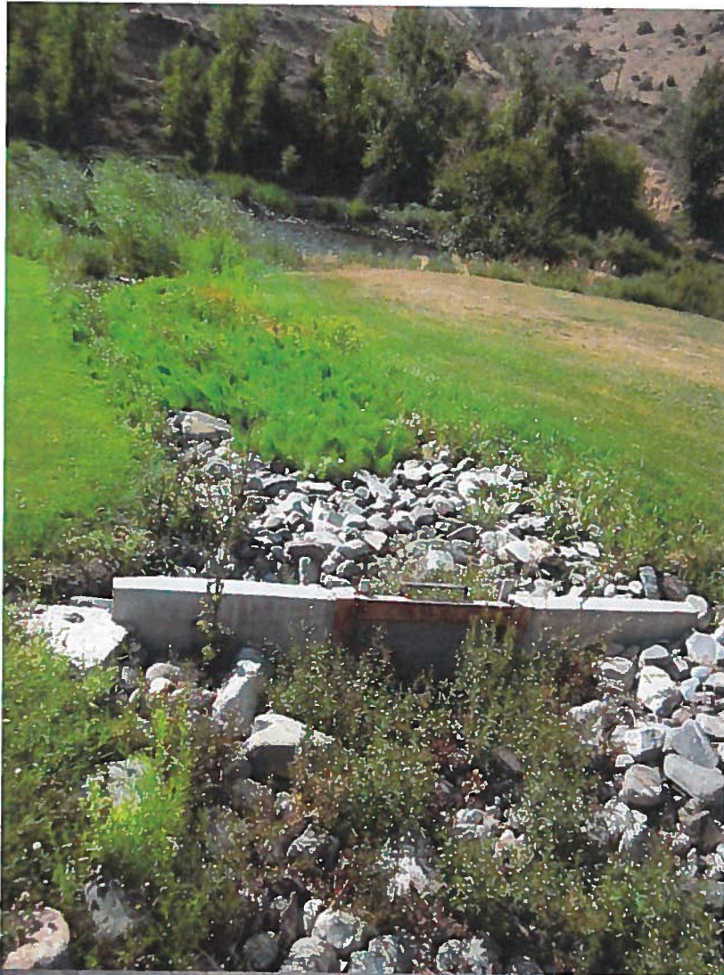
Headgate and channel looking downstream from the pond toward the Salmon River
