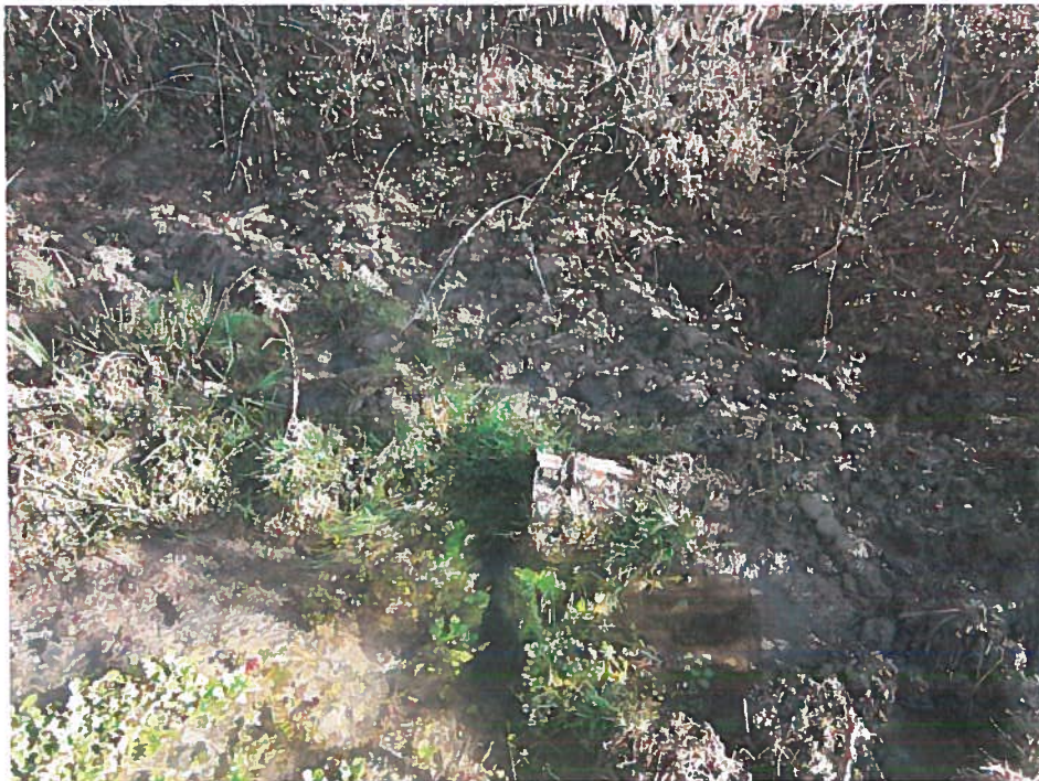
Figure 4: Partially buried 16" pipe, point of diversion from unnamed stream into ditch
