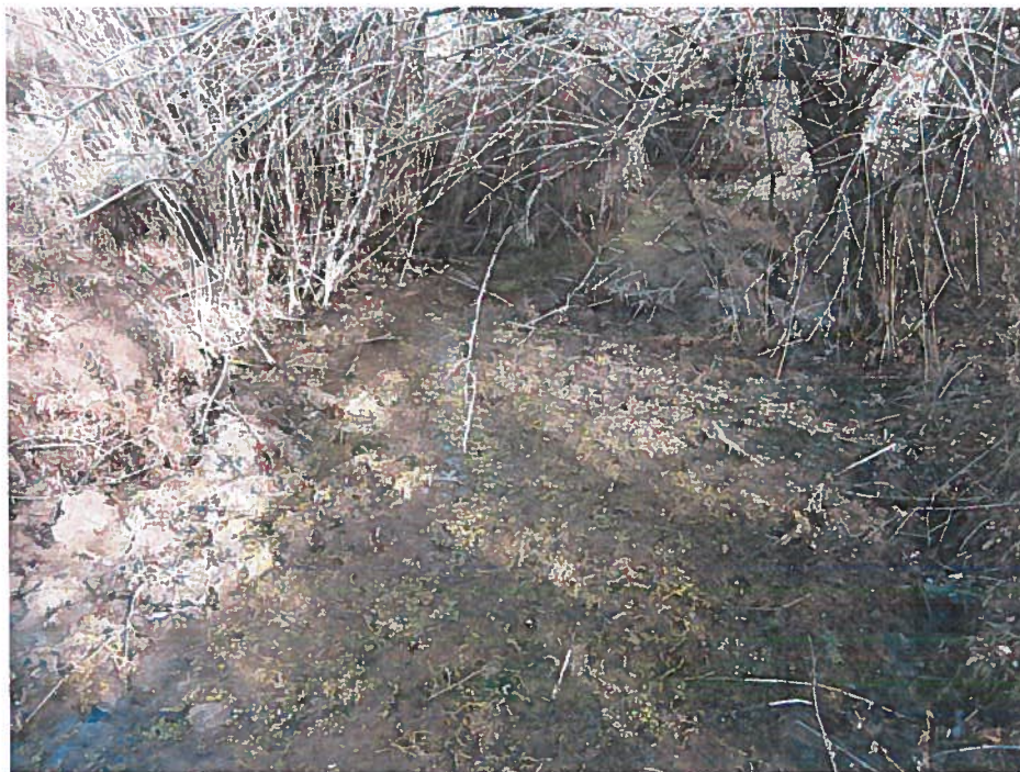
Figure 4: Current state of ditch
