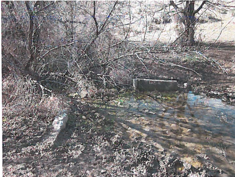
Figure 5: Remnants of check structure on unnamed stream 10' downstream of point of diversion
