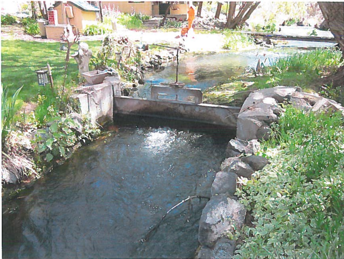
Figure 2: Headgate on Padgett ditch
