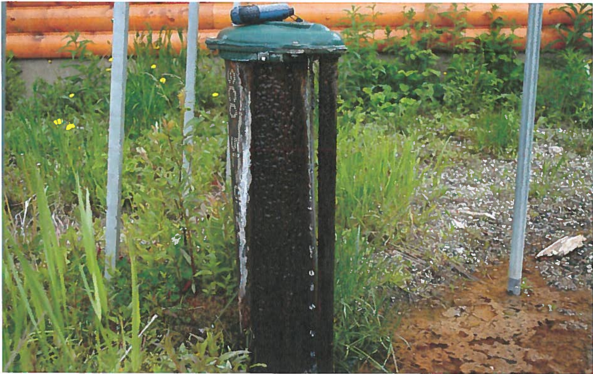
Leaking wellhead
