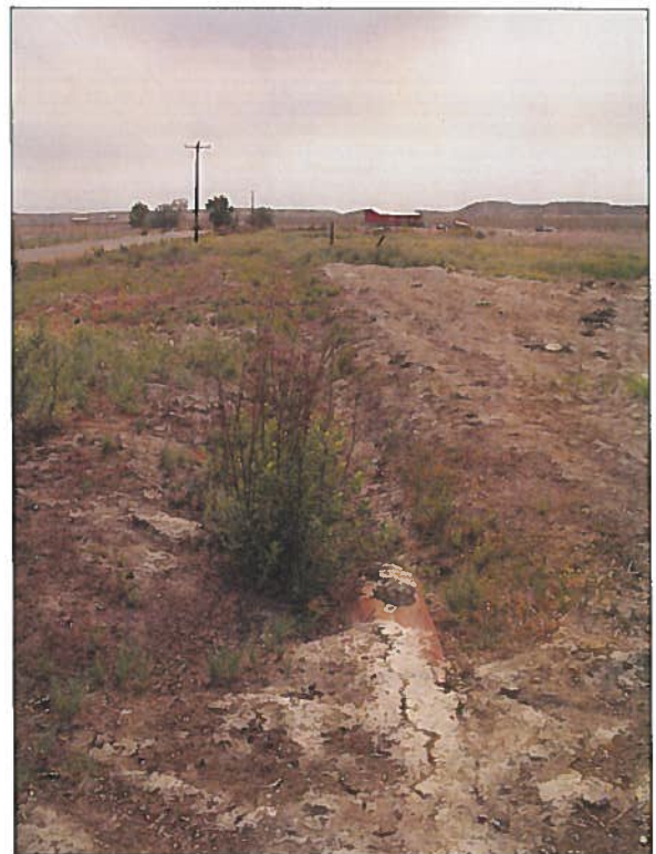
Existing culvert road crossing along the East Side Ditch..
