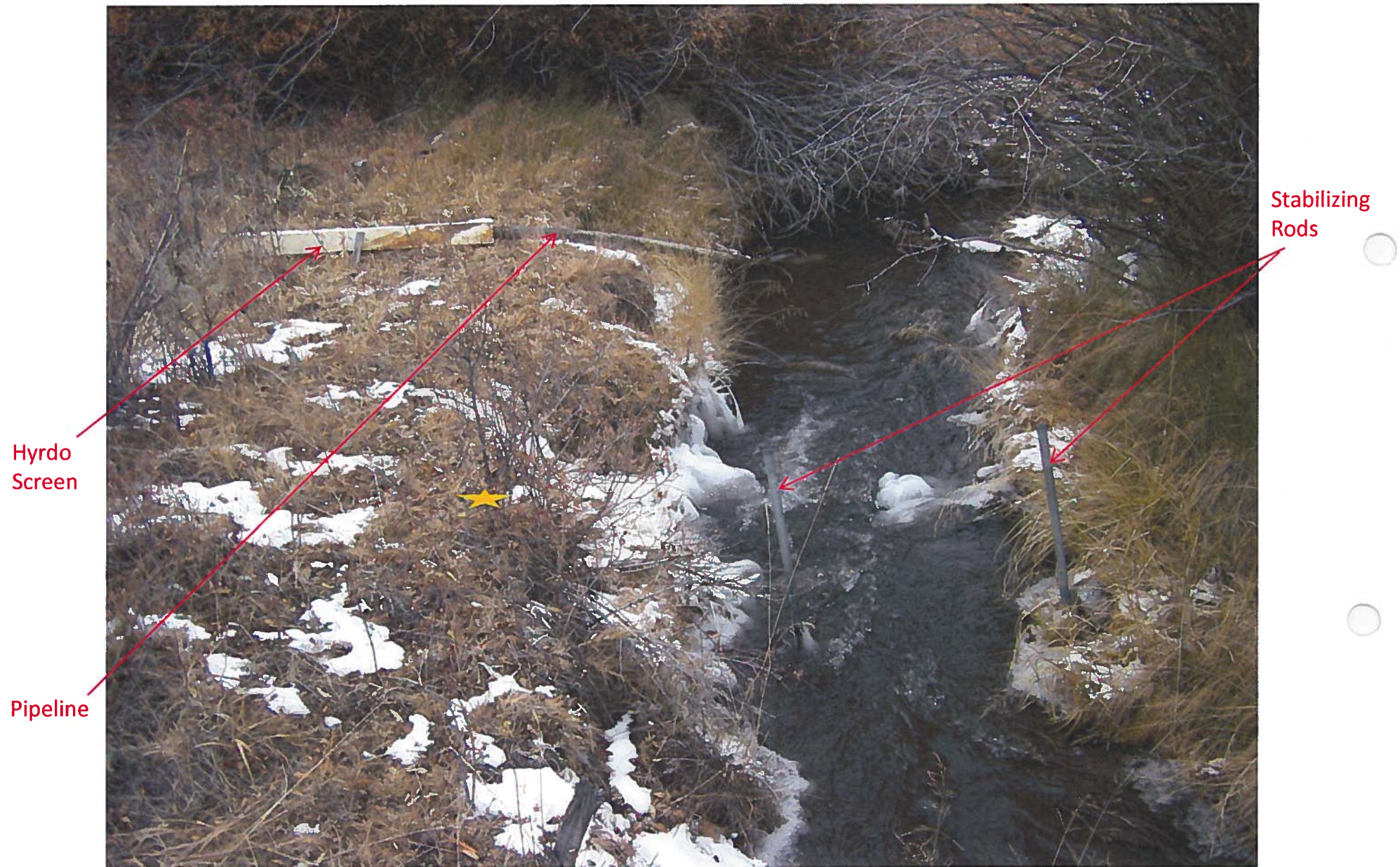
POD, Bert Creek T11N, R24E, S20, NWNW ★ N44.1869 W113.6482 (GPS)
