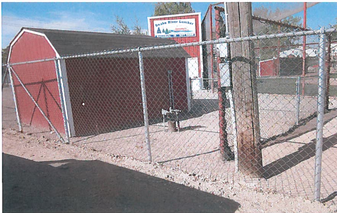
Looking northwest at the well that is the POD.
