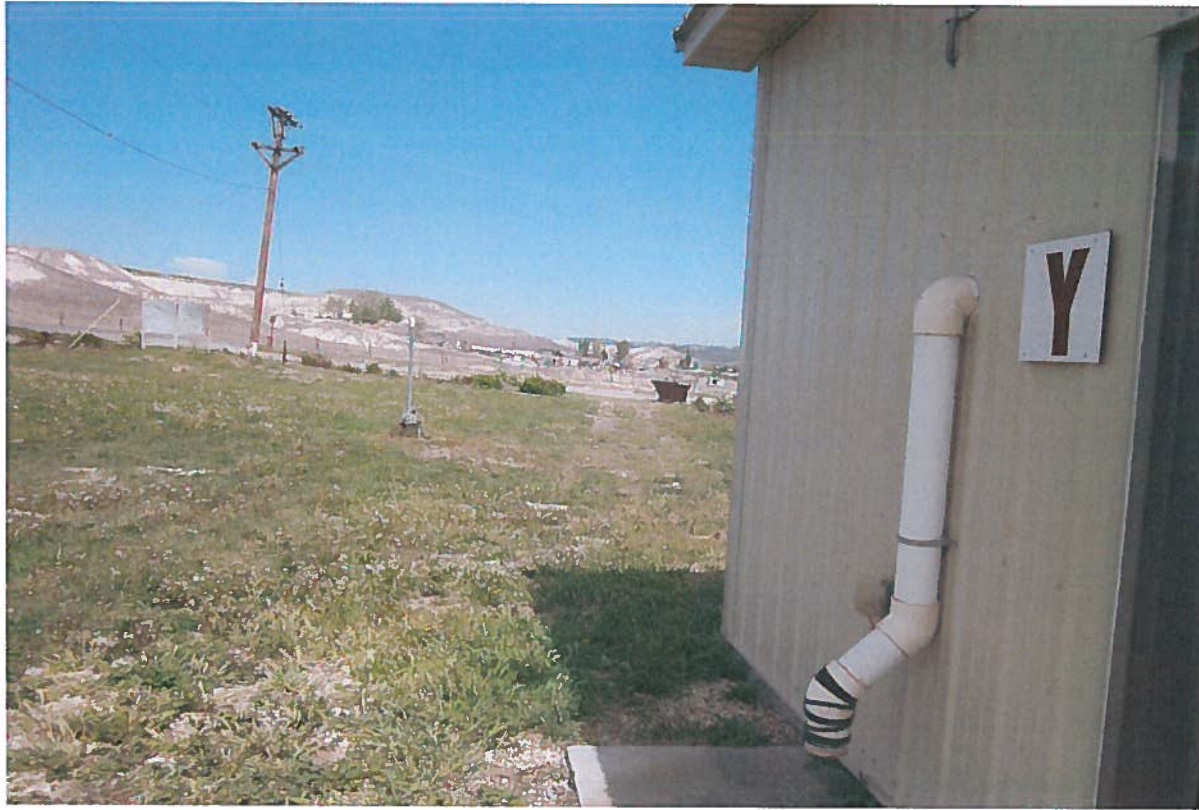
The building labeled "Y" is the pump house. View is looking north at the well.
