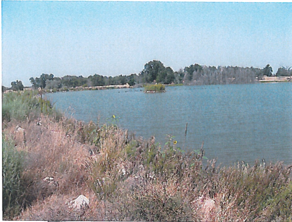
Looking northerly at the reservoir
