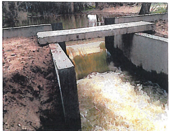
4 – foot rectangular contracted weir with staff gage (on bulkhead) and stilling well (for monitor equipment) placed in ditch above reservoir, near park office.
