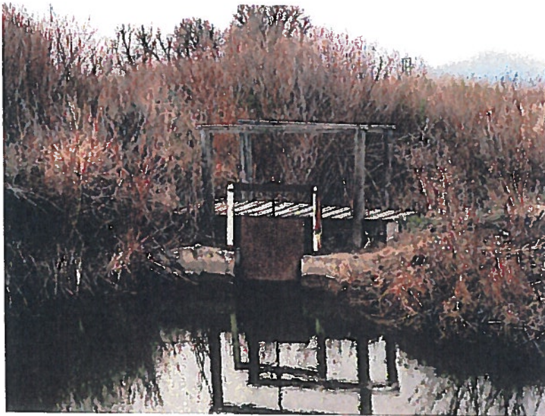
Screw-type control headgate at head of diversion ditch from W- drain.
