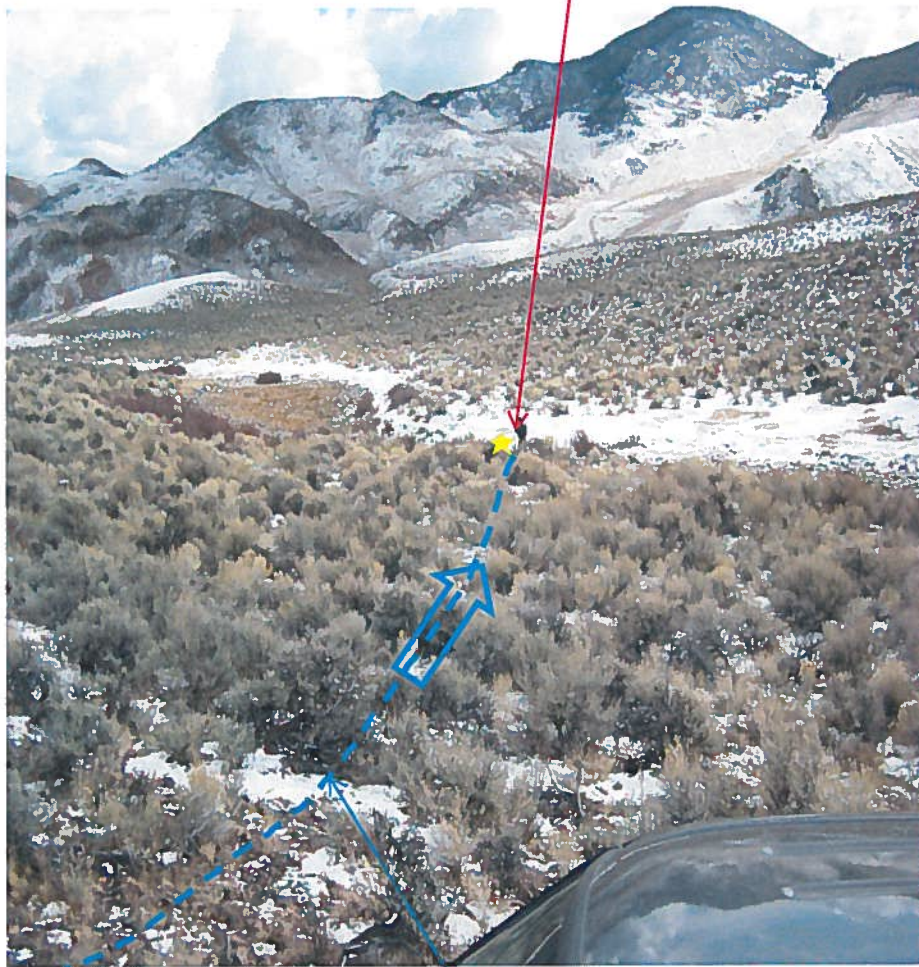
Drain Valve #1 Picture #18 10/25/2012
