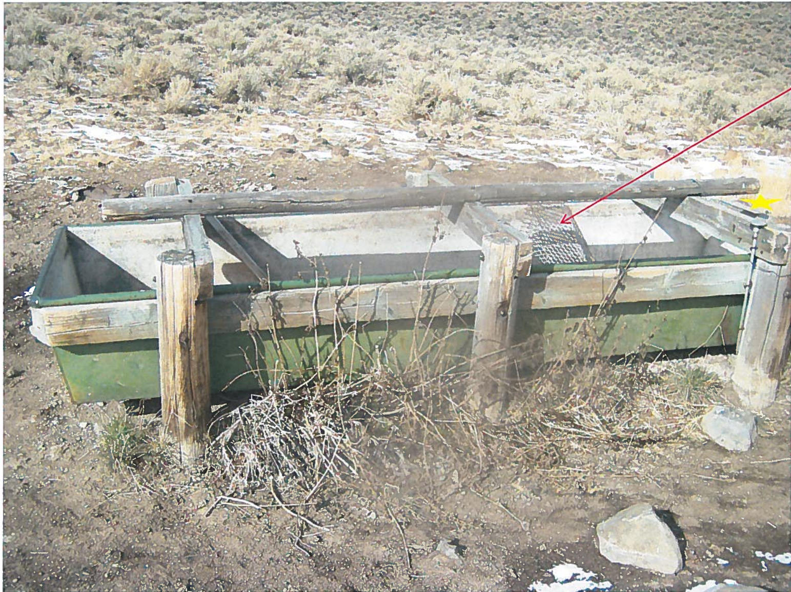
BLM Trough #1 T13N, R22E, S19, NESW ★ N44.4398 W113.9052 (GPS)
