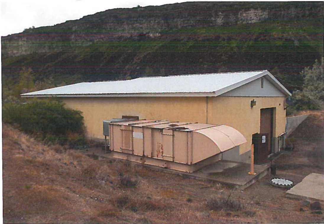
Building housing the hydropower turbines
