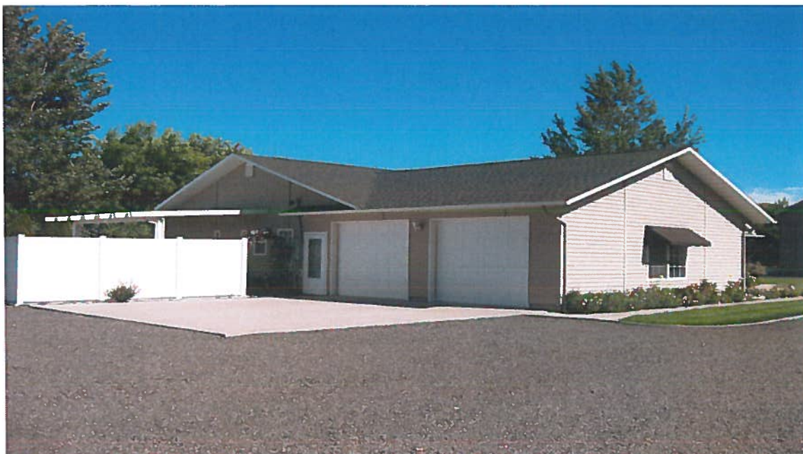
North end of Residence
