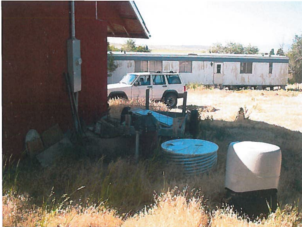
63-31191 Exam 6/18/2013: POD and pump house with mobile home in background facing south.
