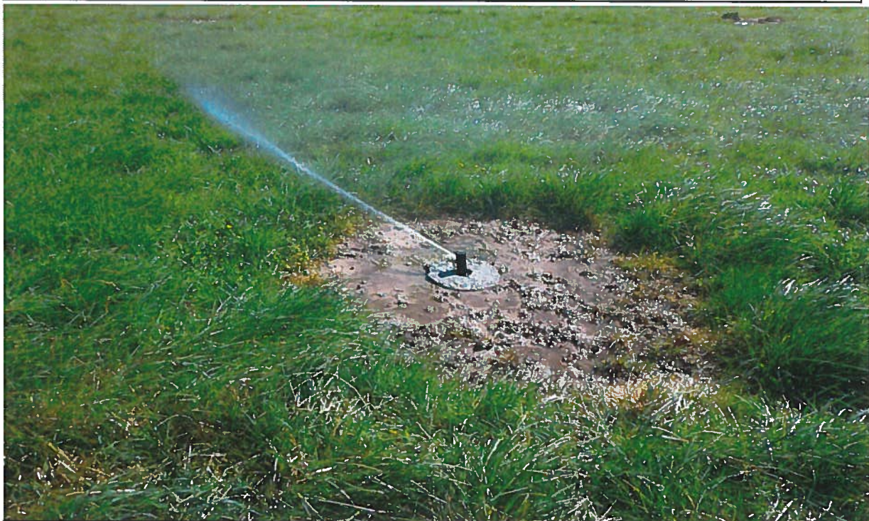
View of a typical Hunter pop-up rotary sprinkler within a concrete collar to protect from livestock damage.
