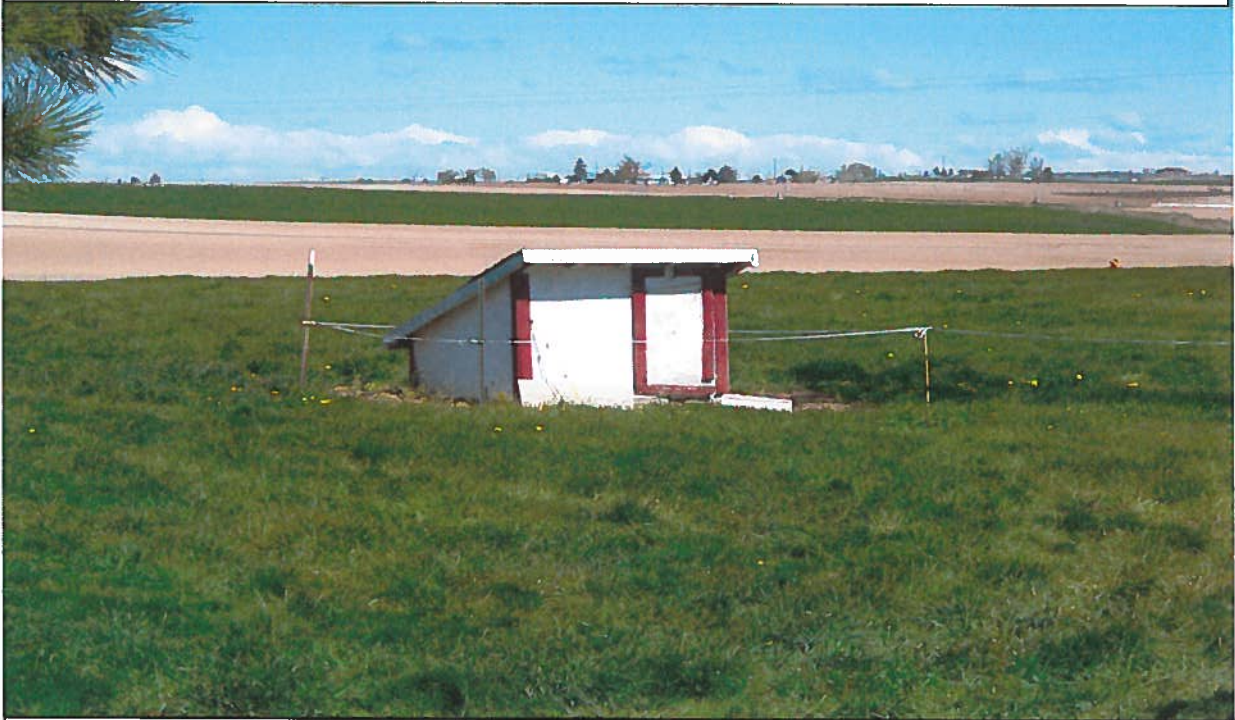
Point of Diversion: View northerly of the well pump house.
