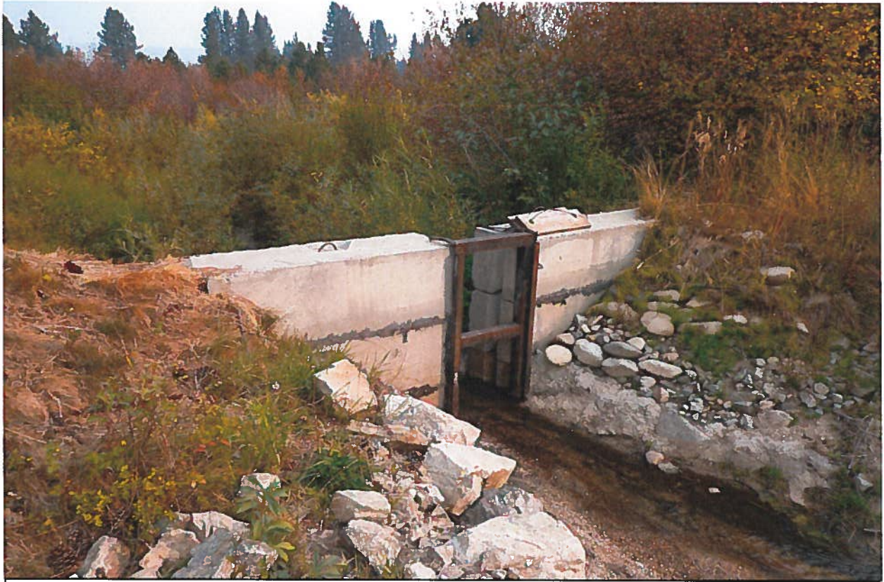
View upstream of concrete dam, slotted channel, and boards used to check up water.
