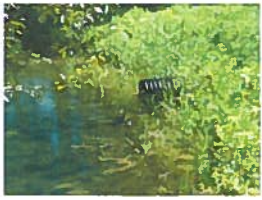
Water Level at Invert of CHDPE.JPG
