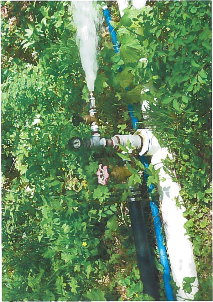
IRIGATION "2" 2" Line Black Pipe
