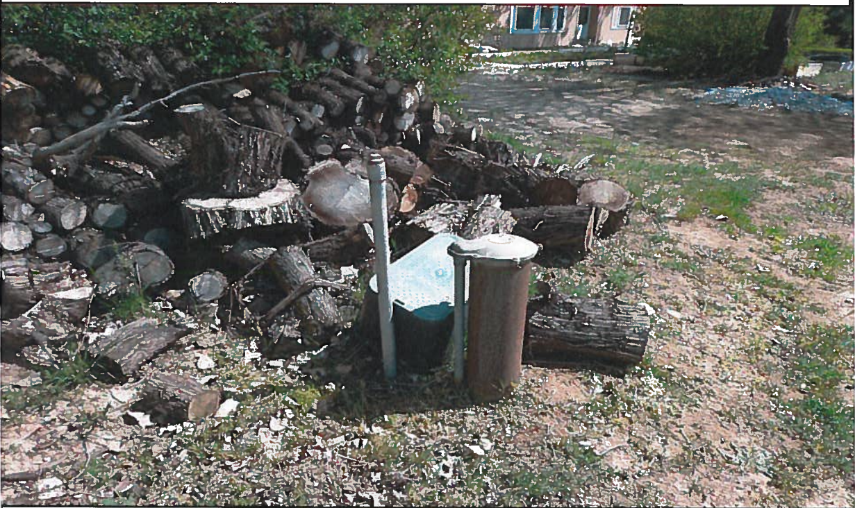
Point of Diversion: View southeasterly of original well serving the Country Corners Campground. The 3" discharge line 'tees' into the main 3" discharge line to the three pressure tanks in the mechanical room of the office building.
