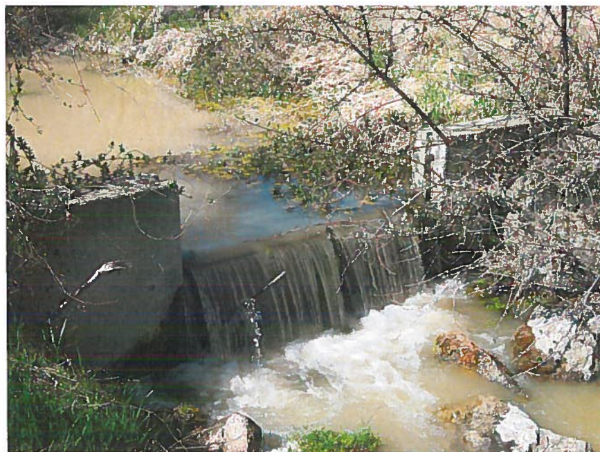
Figure 2: Point of Diversion; Check Dam on Gulch
