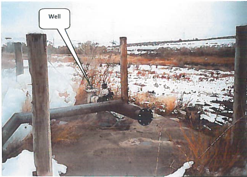
LEFT: View on December 2, 1992 of the well that serves as the point of diversion for right 47-7520.
