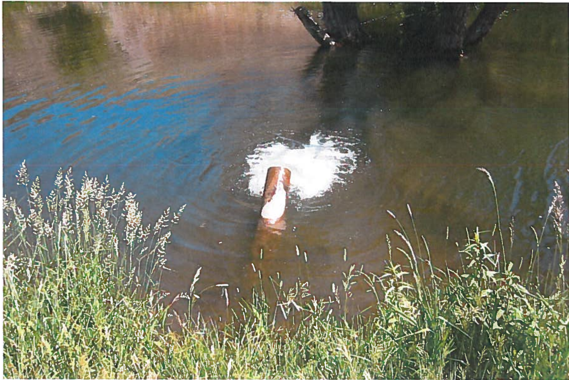
Diversion into series of ponds
