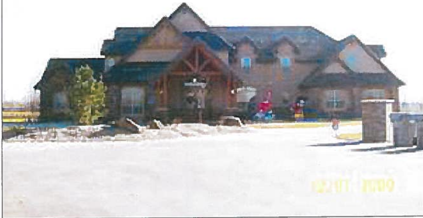
Water utility connection supplied for home built in Rivervine Subdivision, Block 2, lot 21.
