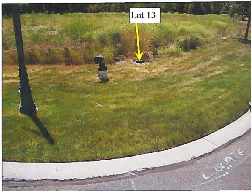
Water utility “stub-ins” for Rivervine Subdivision, Block 1, lot 13.
