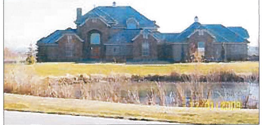
Water utility connection supplied for home built in Rivervine Subdivision, Block 2, lot 22.
