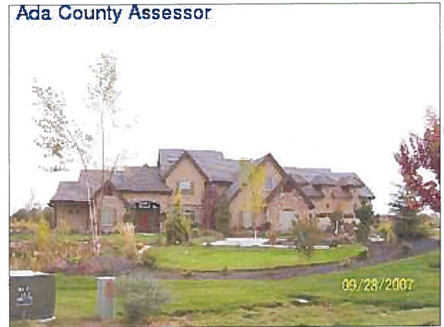
Water utility connection supplied for home built in Rivervine Subdivision, Block 2, lot 20.
