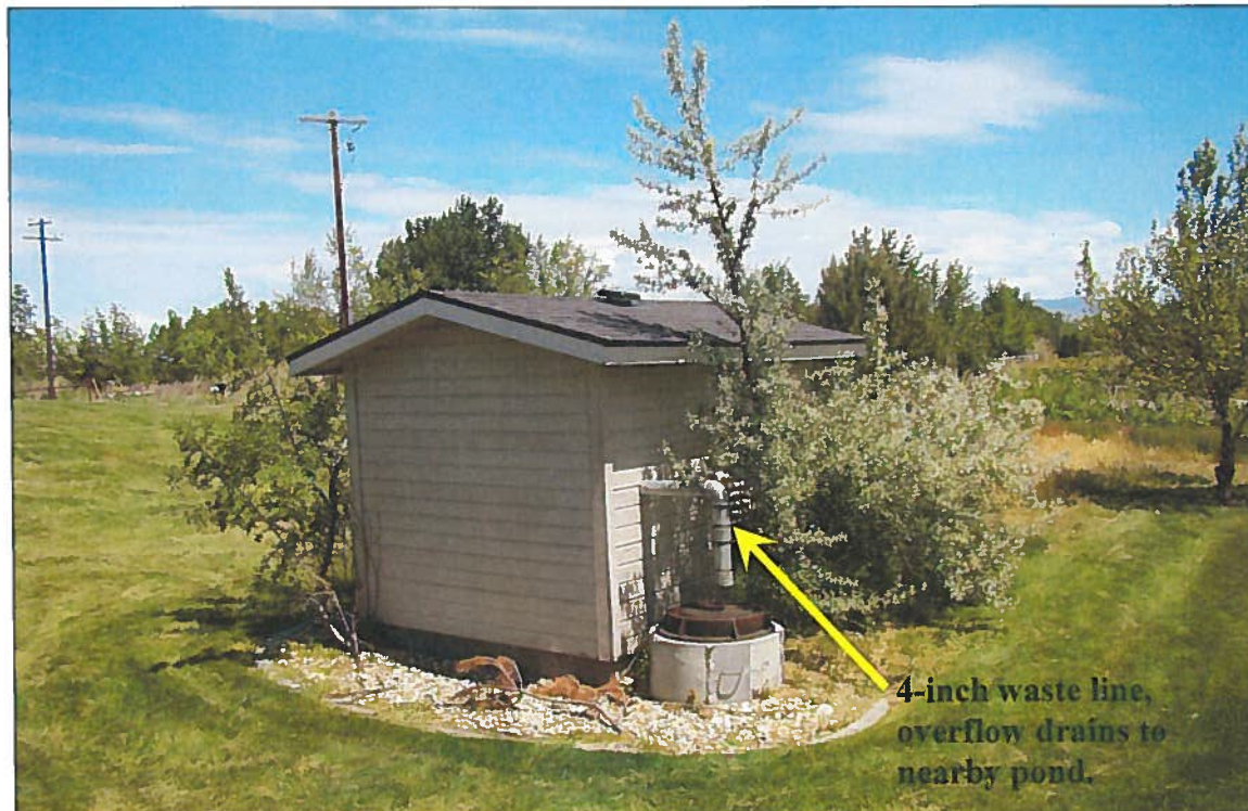
b) Photo looks northeast at Well #1 pump house.
