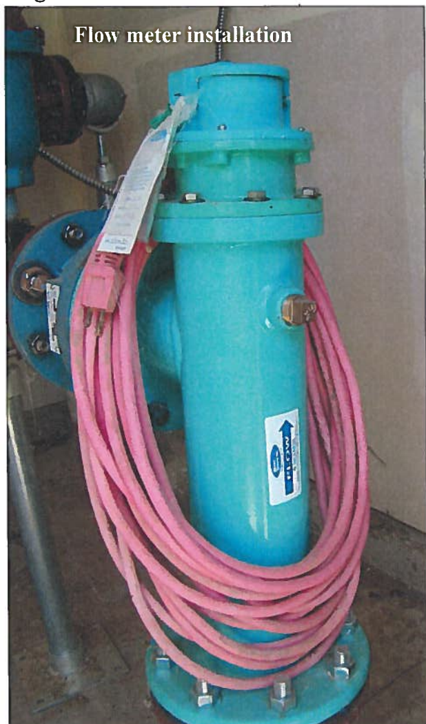
Figure 3. Photos of the 4-inch flow meter and line-pressure gauge for Rivervine Supply Well #1
