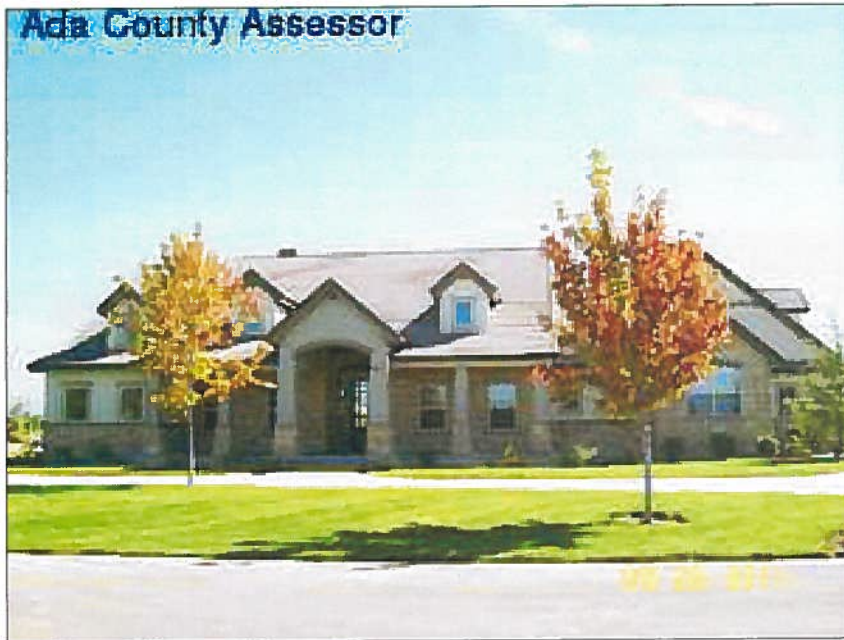
Water utility connection supplied for home built in Rivervine Subdivision, Block 2, lot 19.
