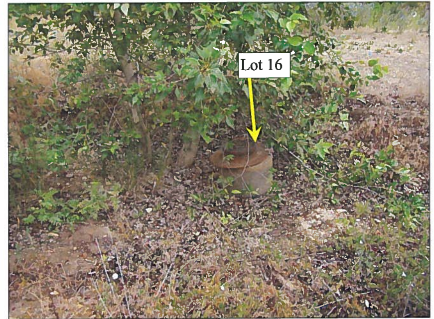
Water utility “stub-ins” for Rivervine Subdivision, Block 1, lot 16.
