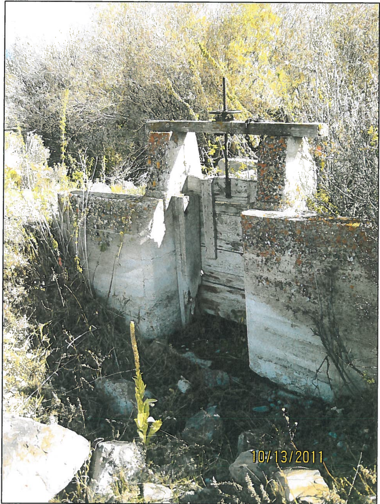
Photo 3b. Historical headgate from the Pahsimeroi River
