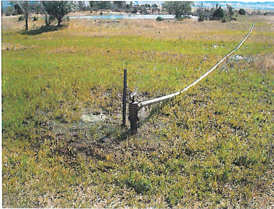
SMT Investors/Scheff Complaint 6/6/2012: Pipe connected to riser off mainline from well draining into far west pond in series of ponds (facing east). Location 10 on map.
