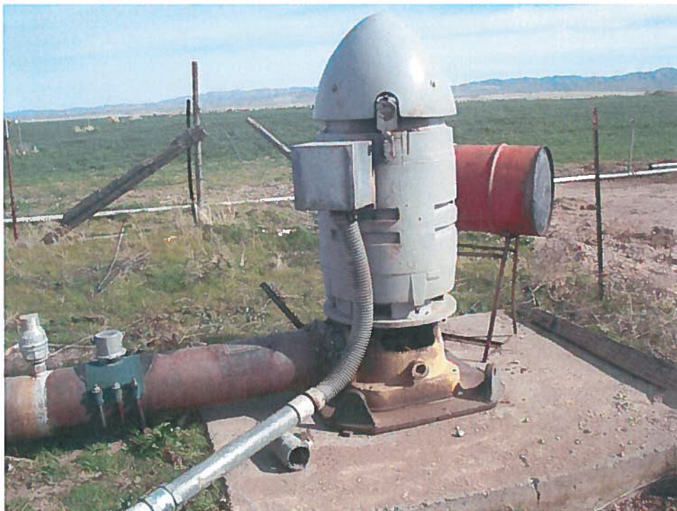
SMT Investors/Scheff Complaint 4/13/2012 Photo #4: Well #1 facing north. Dysfunctional flowmeter on discharge pipe on left side of photo.
