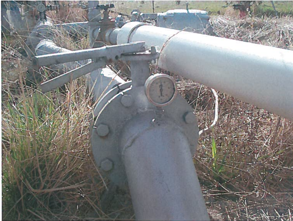
SMT Investors/Scheff Complaint 4/13/2012 Photo #3: Well #2 diversion system facing east. 8" pipe to mainline going into ground. Booster pump and well in background. PVC pipe in upper right of photo goes to buried 1,000 gallon storage tank for house.
