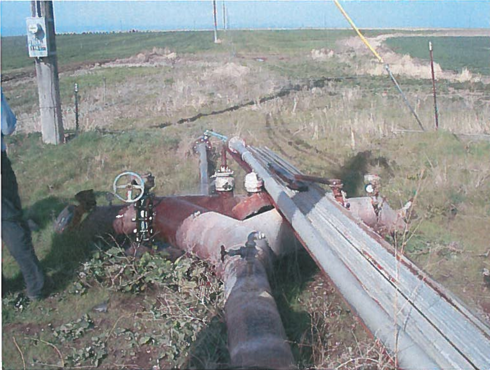
SMT Investors/Scheff Complaint 4/13/2012 Photo #5: Well #1 diversion system facing west. 10" discharge pipe from well in foreground of photo to 12" manifold that splits diverts water to mainline north (right) to pivot and mainline south (left) to risers for handlines.
