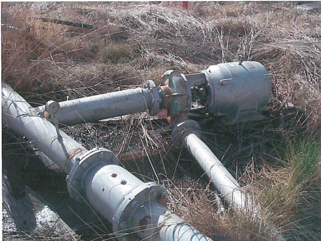
SMT Investors/Scheff Complaint 4/13/2012 Photo #2: Well #2 booster pump facing southeast. 8" pipe to mainline on left side of photo.
